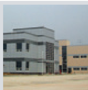
Wuxi Plant (China)
